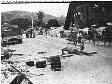
SAPPERS PREPARE A BRIDGE FOR DEMOLITION IN SOUTH JOHORE
