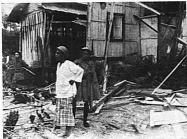
A MALAY A.R.P. WARDEN INSPECTING SOME AIR-RAID DAMAGE
