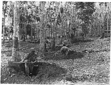
AUSTRALIAN TROOPS DIGGING TRENCHES IN A RUBBER PLANTATION
